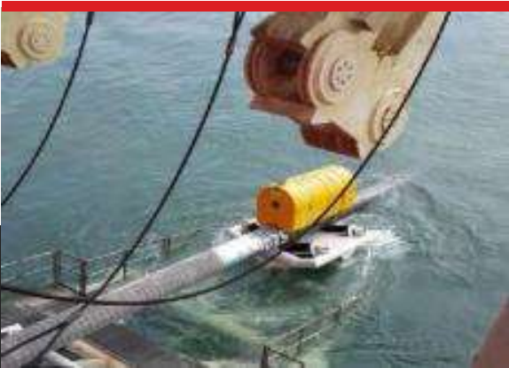
PIPE DEPLOYMENT FLOATS – TIE IN
