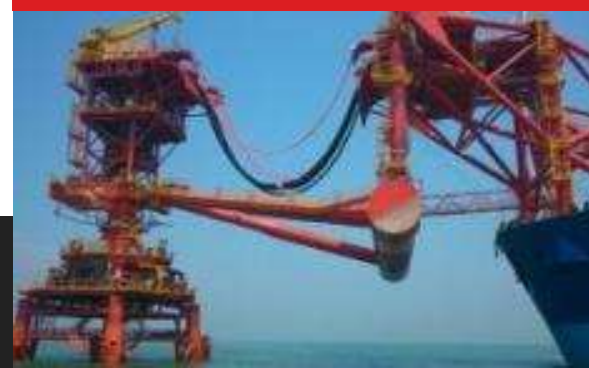
FPSO SWIVEL LOAD MONITORING
