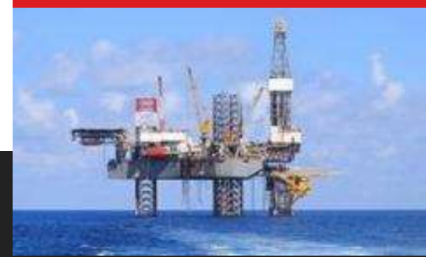
JACK-UP RIG LEG MONITORING
